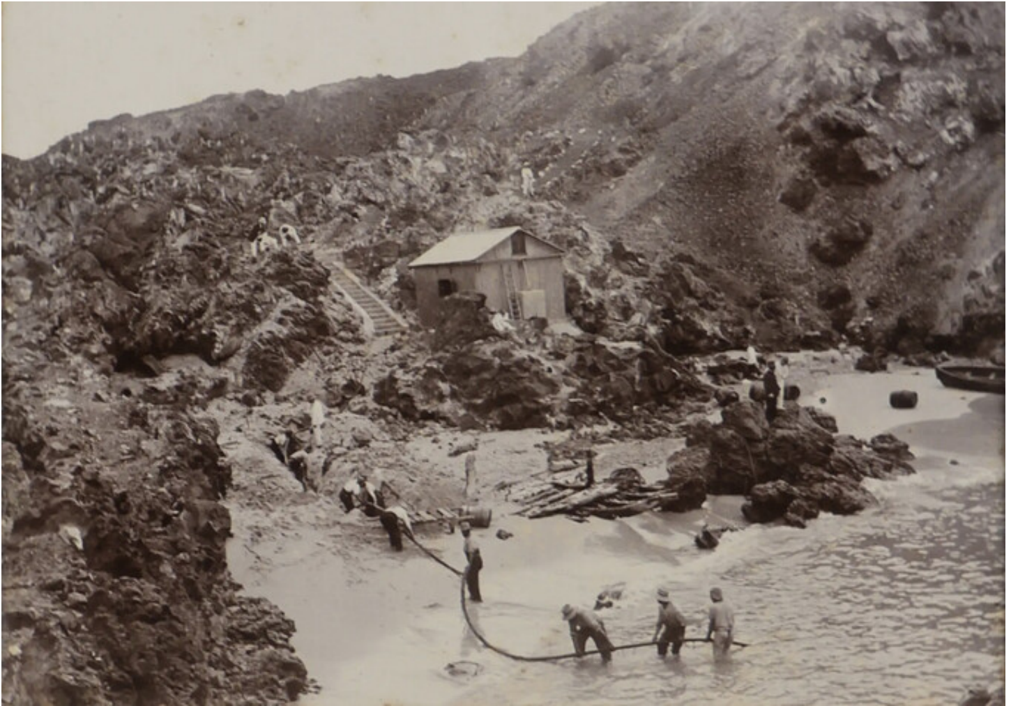
Photograph by Montgomery Williams depicting the laying of cable for the Western Telegraph Company on Ascension Island in 1910.
